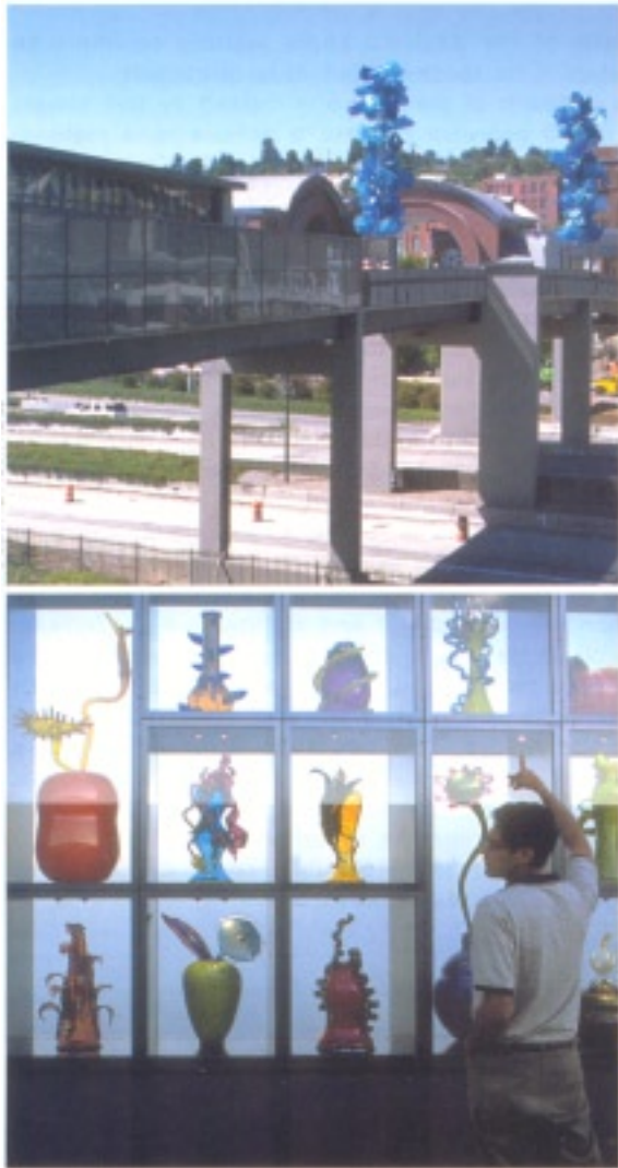
The Crystal Towers (facing page and top left) provide Tacoma with a new landmark. The bridge columns extend 6 to 17 feet above the deck to become the support casings for the pavilions. The display cases are fabricated from blackened stainless steel with a sat-in reflective finish. The Seaform Pavilion (above) allows visitors an intimate experience with the artwork. Visitors are not allowed to “see” the glass until they enter the pavilion, where they are met with an explosion of color and form. In the Venetian Wall (left), selections from Chihuly’s Venetians, Ikebana and Putti series are illuminated with natural light and a fiber optic system.
